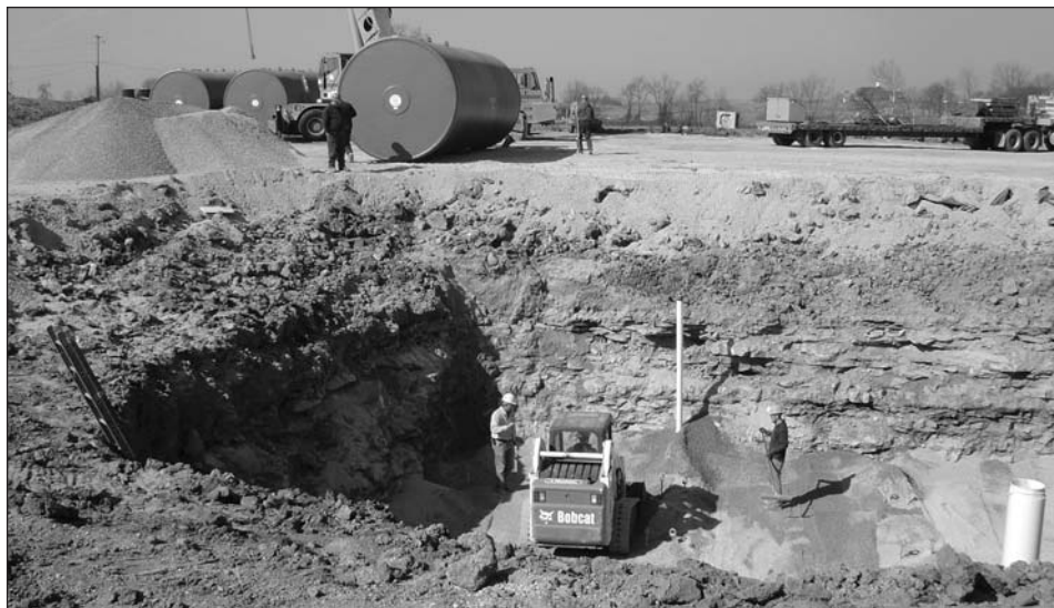
Installation of an underground storage tank in Kentucky. Photo by Division of Waste Management
