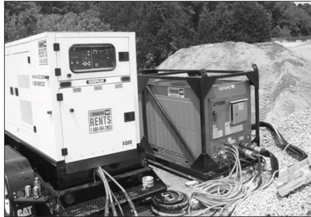
FAR LEFT: Workers with Schnabel Engineering perform a balancing act while tying steel panels for a well form prior to pouring concrete.
