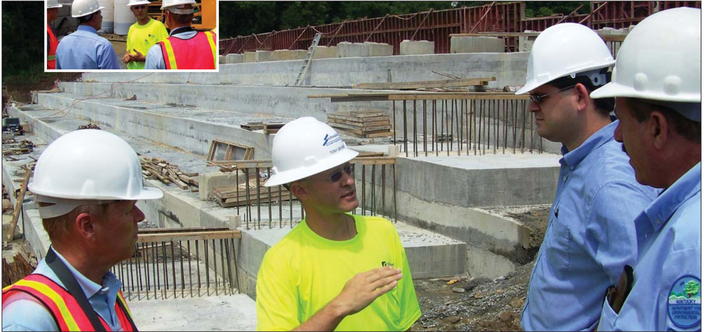
TOP and ABOVE: Tony Grubbs (center) with Schnabel Engineering LLC describes the process of producing roller-compacted concrete in the rapid mixer facility and explains the stepped dam design to DOW engineers (from left) Gary Wells, Glen Alexander and Mortaza Rabiee.
